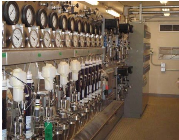
Figure 2: Sample Panel Day before Starting HRSG Commissioning
