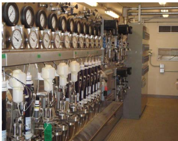
Figure 2: Sample Panel Day before Starting HRSG Commissioning
