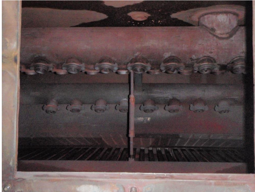
Figure 14: Dual Pipe Inlet Water Distributors
