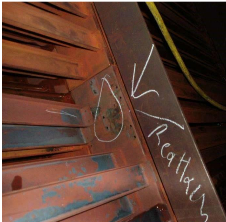
Figure 16: Snapped Top Trays.
